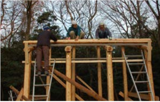
Figure 7, the completed structure of the pillars and roof
