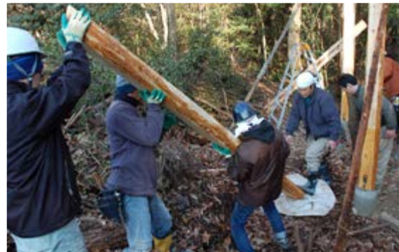
Figure 5, erecting the pillars
